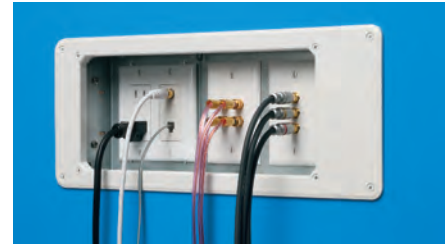
5 Install devices and plates.
