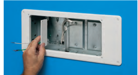
4 Install voltage separator.
