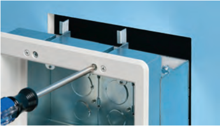
1 Cut hole using enclosure, without trim plate, as a template. (Mounting wings hold box in wall.)
