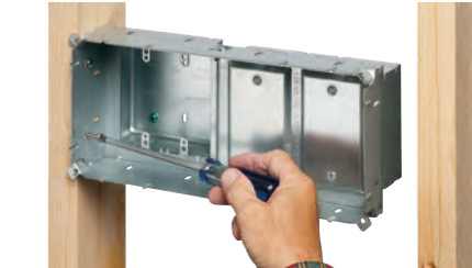
2 Or attach to a wood stud using #6 screws. Pull wires.
