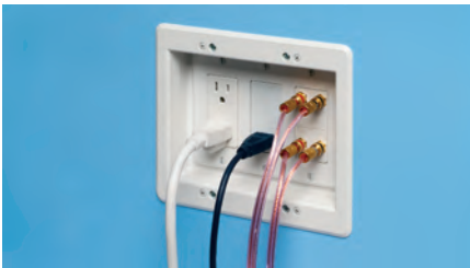
4 Install devices, then the wall plates.
